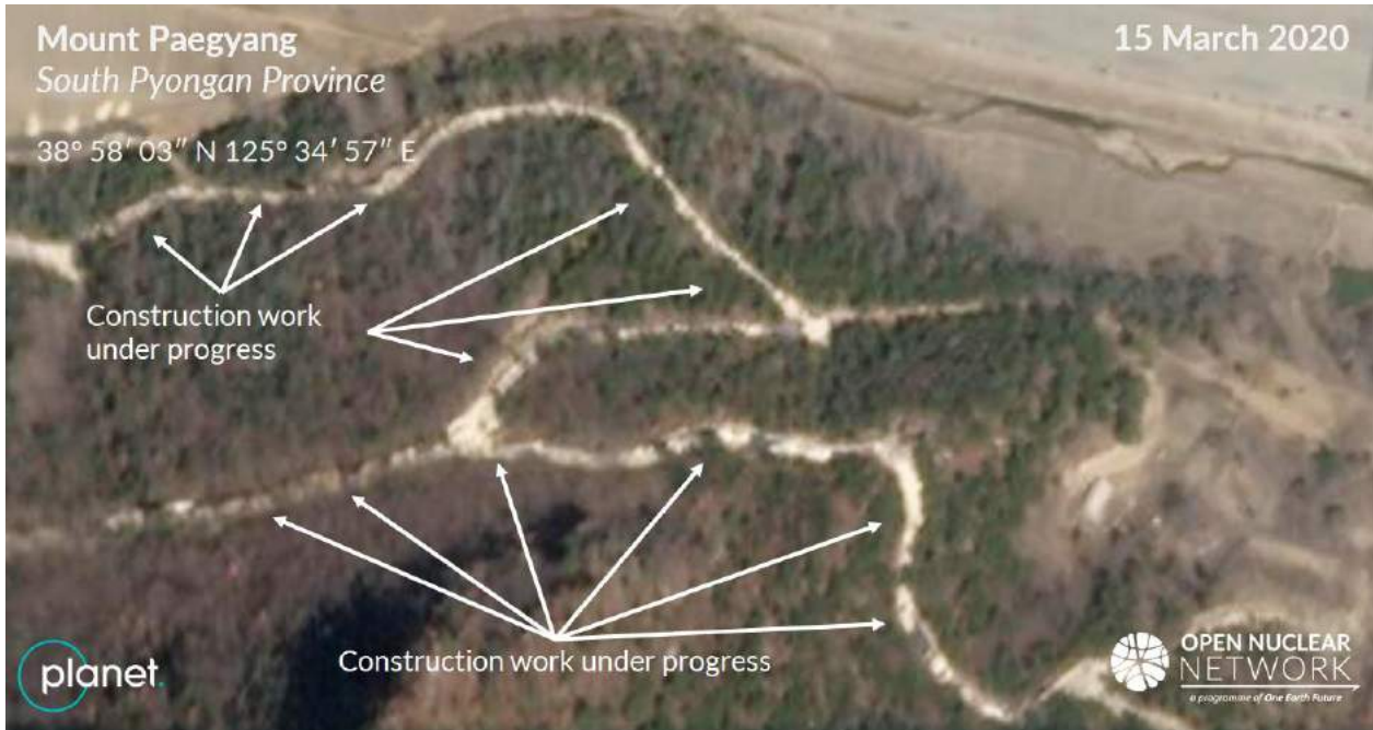
Figure 5. Construction work under progress as of 15 March 2020. Image: © 2021 Planet Labs Inc. All Rights Reserved. Reprinted by permission.
