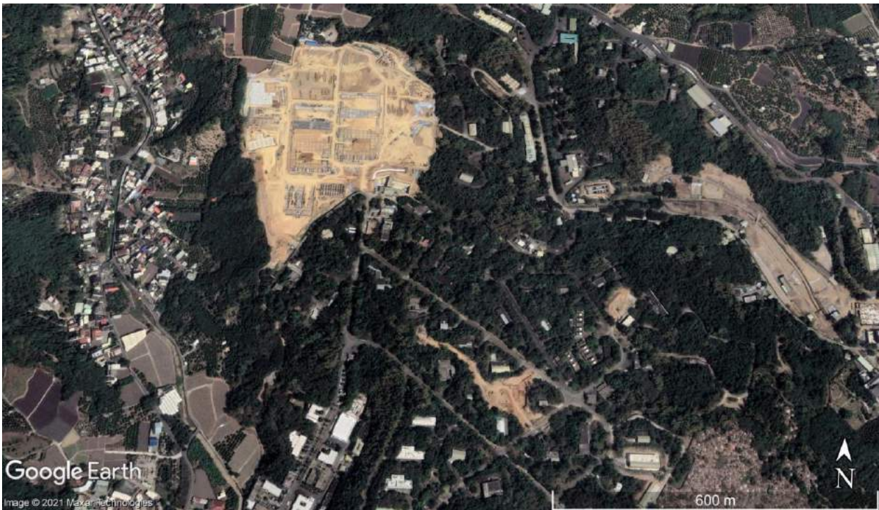
Figure 7. NCSIST Dashu compound, Kaohsiung city. The on-going construction in this February 2021 image comports with media reports that part of Factory 205 will be moved into the Dashu compound. Coordinates: 22°42'3.15"N, 120°25'37.63"E.
