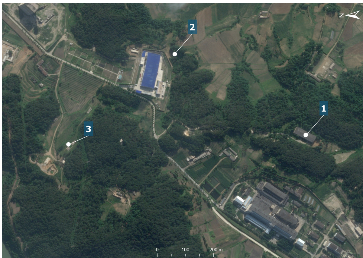
Figure 11: Locations of the three main waste sites. 1 – Building 500; 2 – buried waste site declared to the IAEA; 3 – undeclared old waste site. 27 June 2026. Image: © 2026 Planet
