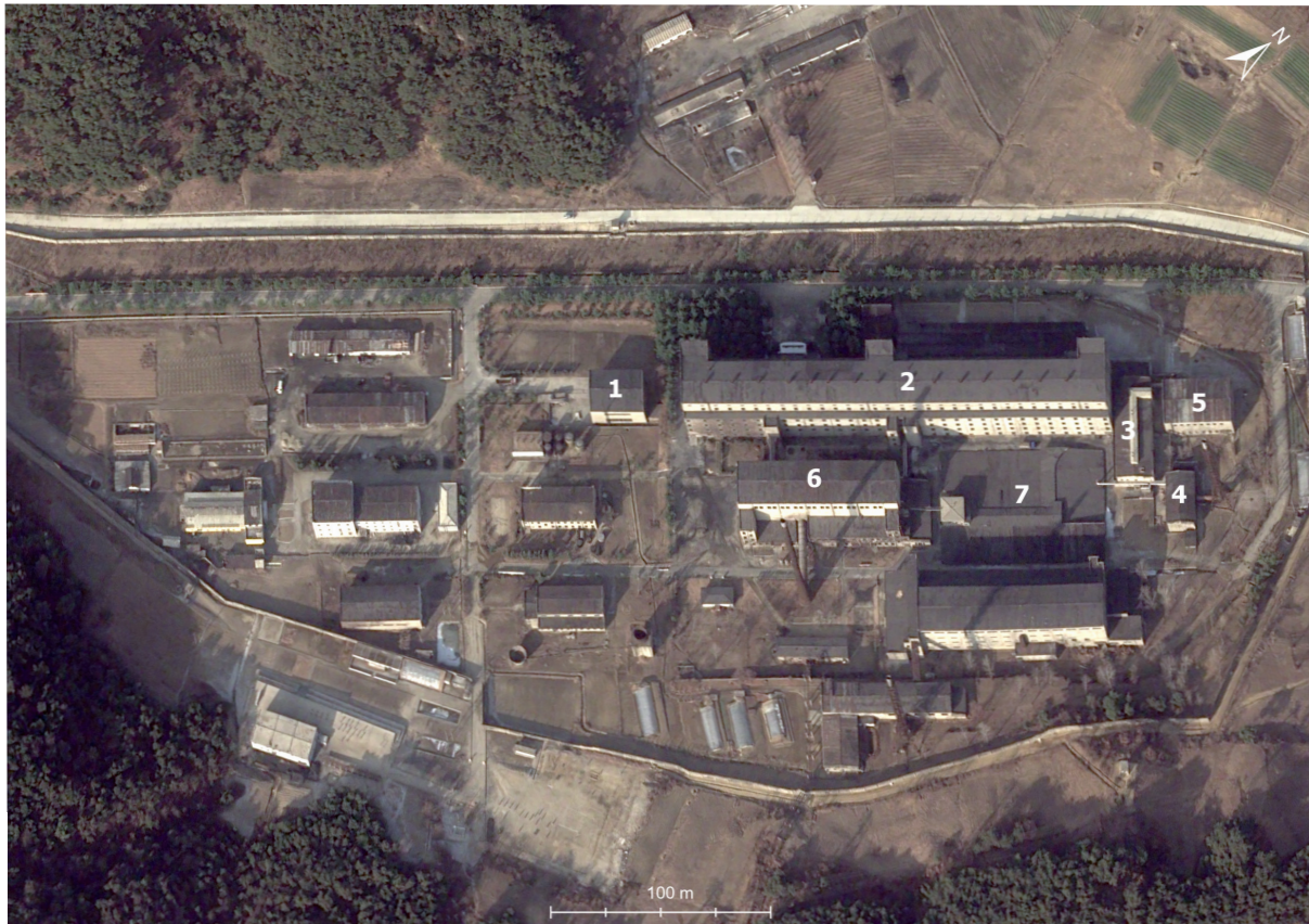
Figure 10: Radiochemical laboratory. 1 – fuel receiving building; 2 – main process building; 3 – metal processing; 4 – off-gas treatment; 5 – washing/decontamination; 6 – high level waste; 7 – low and intermediate level waste. 39.780 N, 125.752 E. 16 December 2025. Image: Airbus DS (2025)
